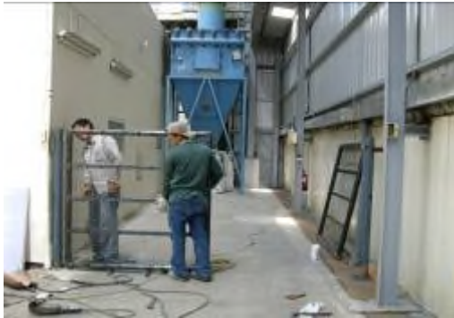
C-0102含鉛集塵灰貯存區無獨立區隔
