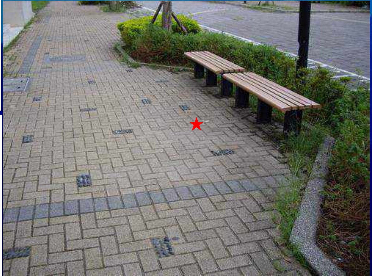
Figure 3.7.4 Space requirements for wheelchairs adjacent seating
