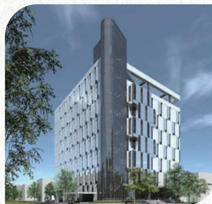
New Phase II standard factory building
