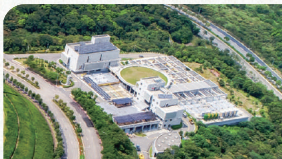
Tongluo Science Park sewage treatment plant
