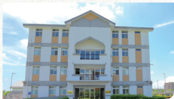
Yilan Science Park sewage treatment plant
