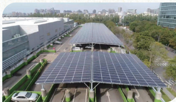
Parking tower at Si-Soft Research Center
